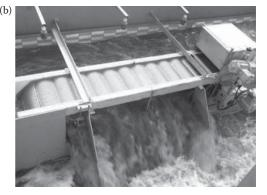
**FIGURE 7.22** Use of special screens for treatment of stormwater or combined sewer overflows: (a) retractable bar screen with trash basket (Courtesy Huber Technology, Inc.), and (b) overflow weir screen (Courtesy John Meunier Products/Veolia Water Technologies Canada).
