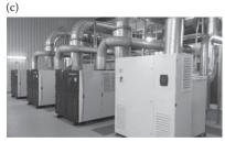
**FIGURE 10.56** Examples of air blowers used for diffused-air aeration systems: (a) positive displacement (Courtesy Aerzen USA Corporation), (b) multistage centrifugal (Courtesy Gardner Denver Nash, LLC), and (c) high-speed turbo (Courtesy Sulzer).
