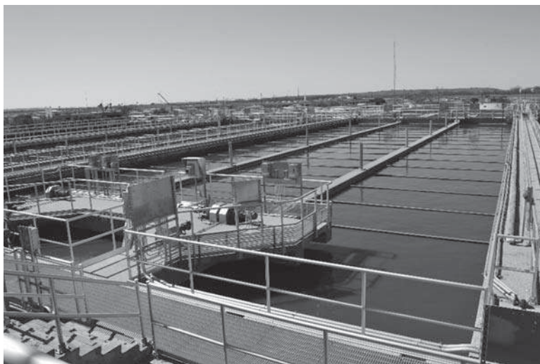
FIGURE 9.6 Rectangular primary sedimentation basins (Courtesy CP&Y, Inc., Dallas, Texas).
