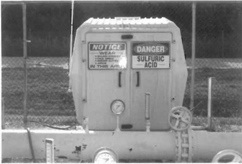
Figure 3.13 In-line addition of sulphuric acid to a recirculating cooling system in St. Petersburg, Florida
